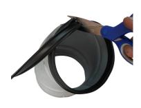
Measure and cut the rubber sealing according to the dimension of the fitting
